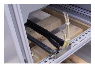
Figure 4-9 Connecting cables in the delivered state (e.g. transport units)
