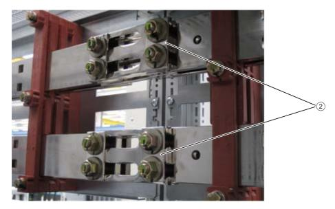
Figure 4-5 Connecting the DC busbar when cabinet units are installed side-by-side
