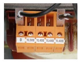
Figure 4-11 Connecting terminals for the fan transformers (2-ph. 380 to 480 V AC)
